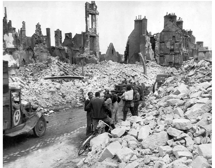
Above: With the rubble cleared from the roadways, the US Army vehicles could pick their way through Valognes on their way north to the battle for Cherbourg. (Photo: US Signal Corps)
