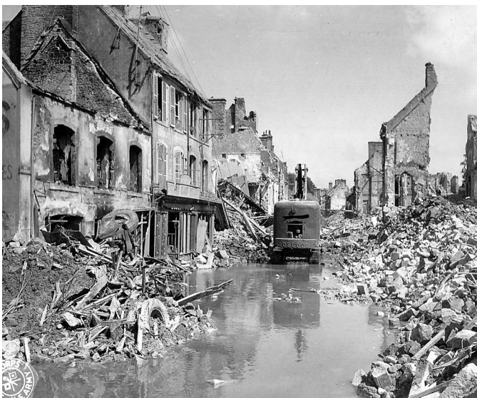
Above: The bombing of Valognes not only devastated buildings, it destroyed infrastructure. Here a water main had burst, while a US Army engineer manoeuvred his Osgood earth-mover. Note the bombed half-house on the right. (Photo: US Signal Corps)
